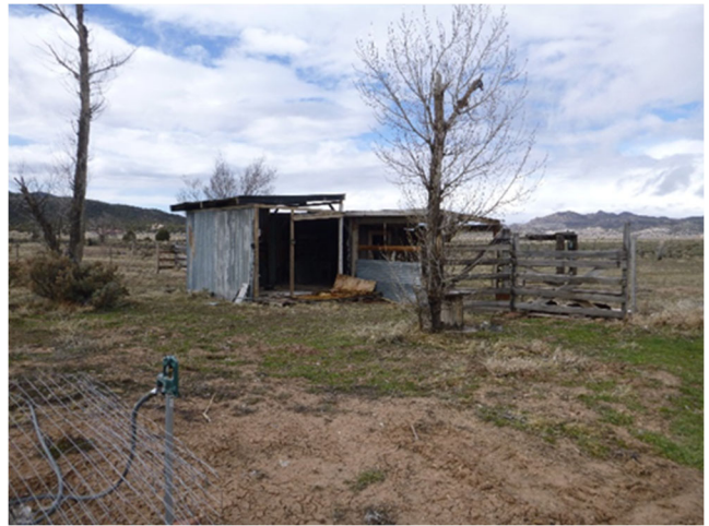
Outbuilding (looking north)
