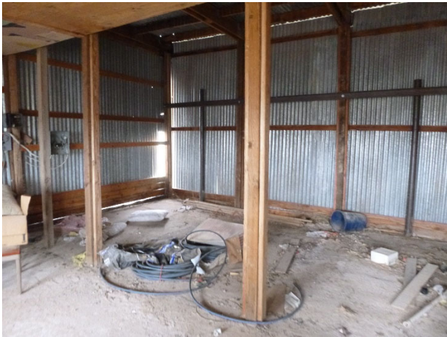
Inside unfinished housing unit
