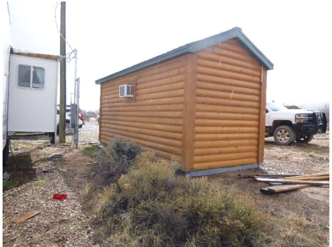
Outbuilding (looking SW)
