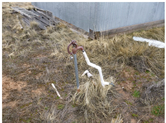
Water spigot near unfinished housing unit
