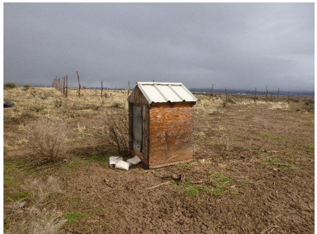
Small structure (looking east)
