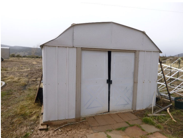
Shed (looking west)
