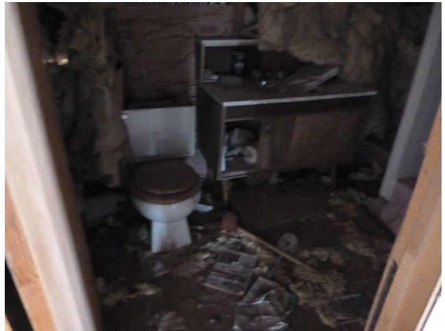
Bathroom inside unfinished housing unit
