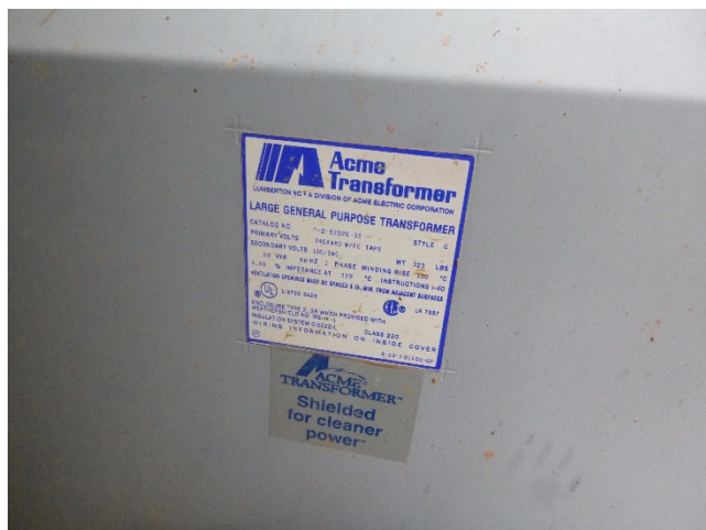
Close-up of well generator
