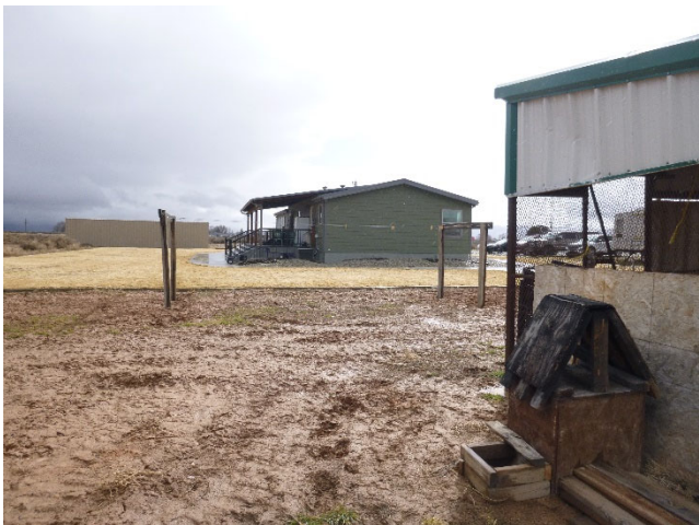
Small shed looking towards house (looking south)
