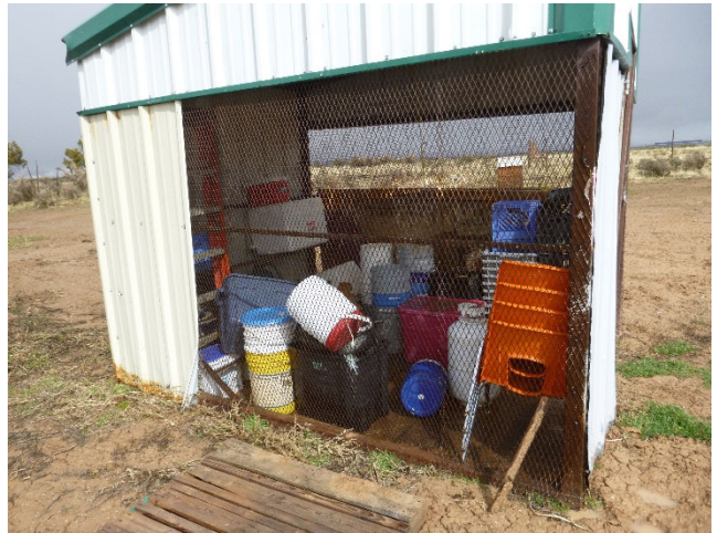
Smaller shed (looking NE)
